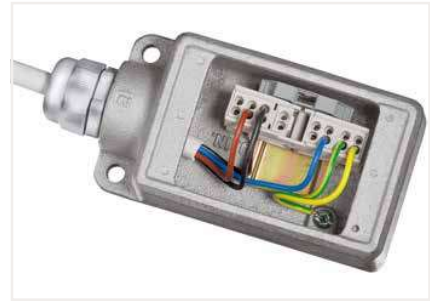
Wiring example in an Ex junction box
