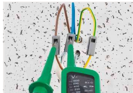
Testing via separate test ports.
